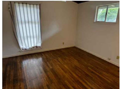
Master bedroom baseboards installed
