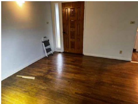
Entry baseboards installed
