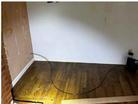
Living room south baseboards installed
