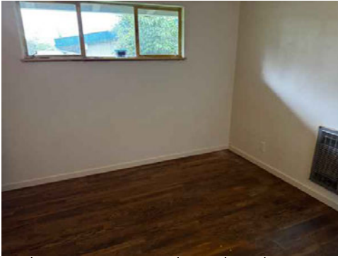
Bedroom 1- receptacle replaced; cover plate installed
