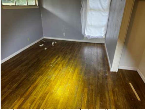
Bedroom 2 baseboards installed
