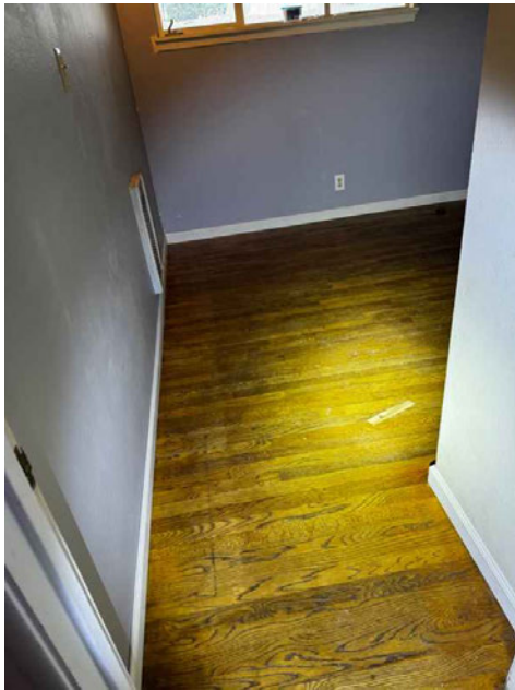
Bedroom 2 baseboards installed
