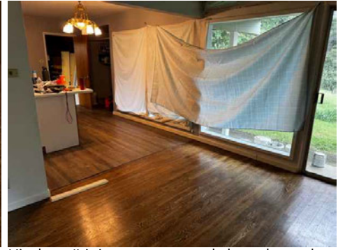
Kitchen/Living room north baseboards installed
