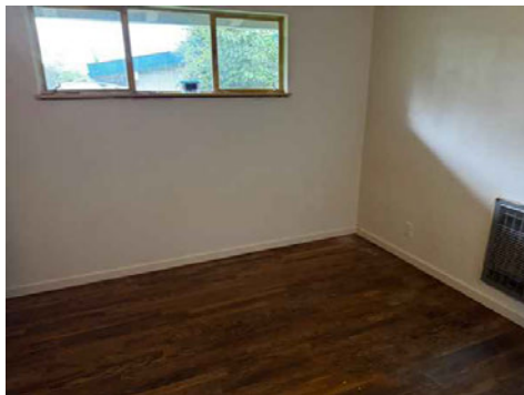
Bedroom 1 baseboards installed
