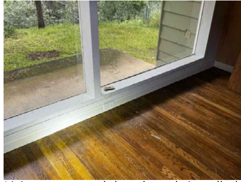
Living room north baseboards installed
