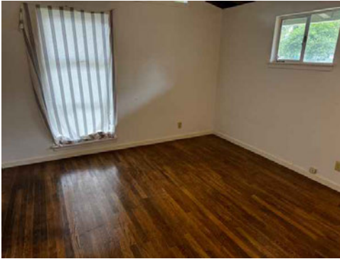
Master bedroom cover plates installed
