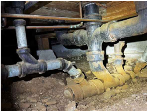
Soil stack with water running: No master tub leaks; no ABS and P-trap replaced as shown on customer invoice
