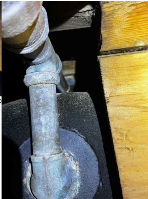
Master tub/shower with running water - no leak; no ABS repairs as invoiced
