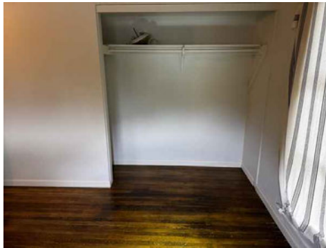
Master bedroom baseboards installed
