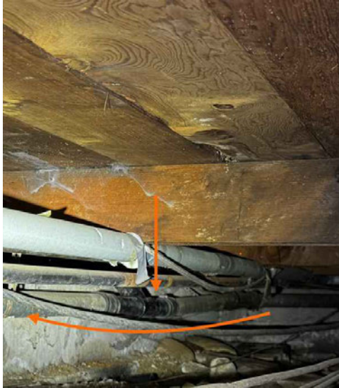
Negative slope at repair site (arrow is direction of flow)
