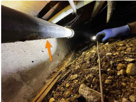
Leak downstream of kitchen sink drain repair
