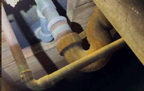
Master tub plumbing (appears original to the home)
