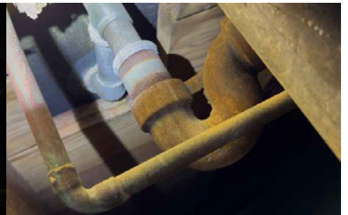
Master tub plumbing (appears original to the home)
