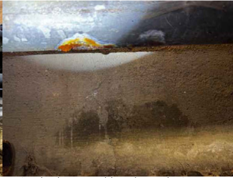
Active leak caused by electrolysis <12" downstream (east) of kitchen drain line repair
